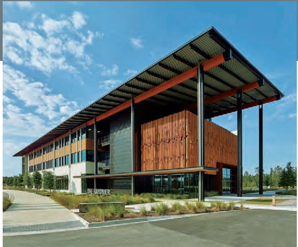
Rayonier Headquarters, photo courtesy of Rayonier
